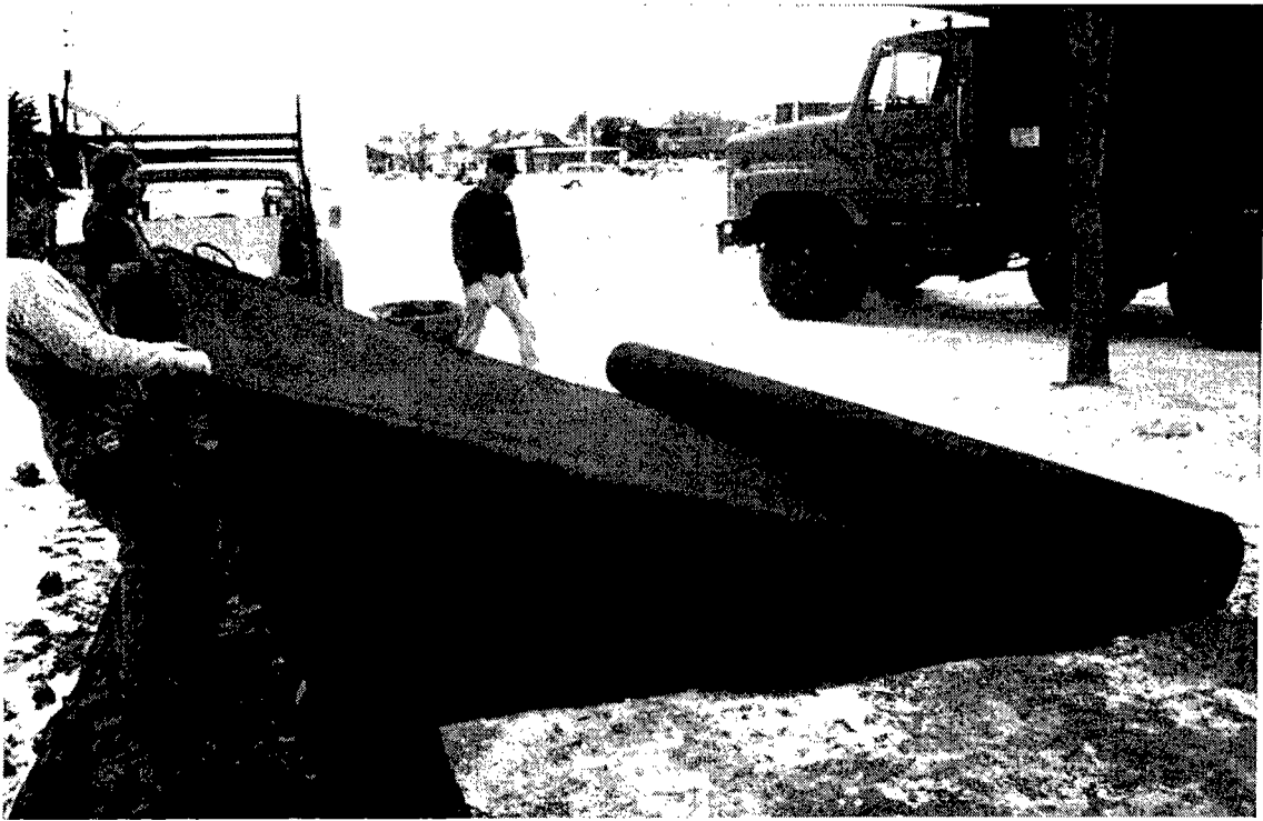
Figure 5.19 Minocqua, WI, MCTT, filter fabric being prepared for installation (WI DNR photo).
